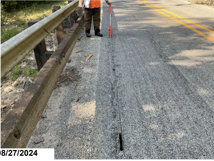
Grout missing between units 6 and 7
