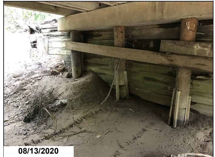
Abutment 2 pile 1 has not been repaired
