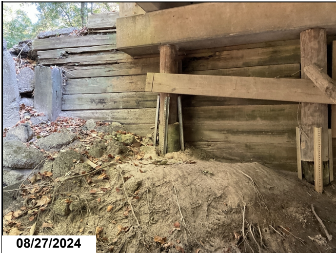
Bent 3 pile 1 has been repaired
