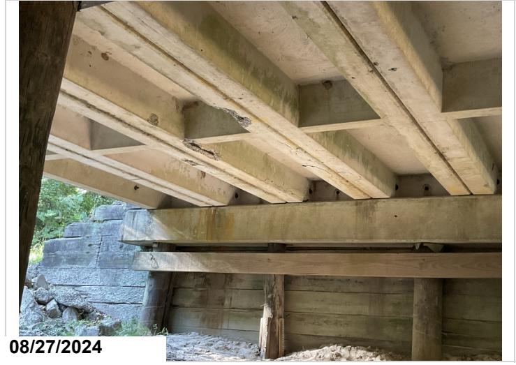
Span 1 units 5 and 6 cracks in legs and spalls with exposed rebar
