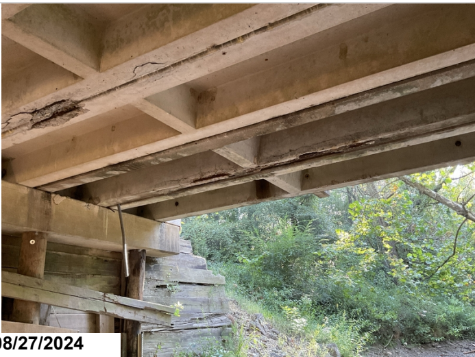
Span 2 unit 6 right leg spall with exposed rebar
